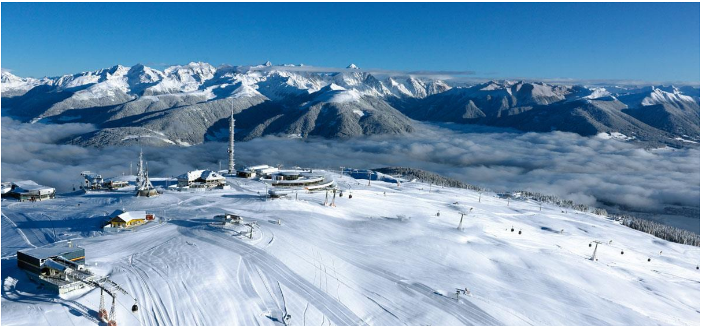
View of Kronplatz top station
